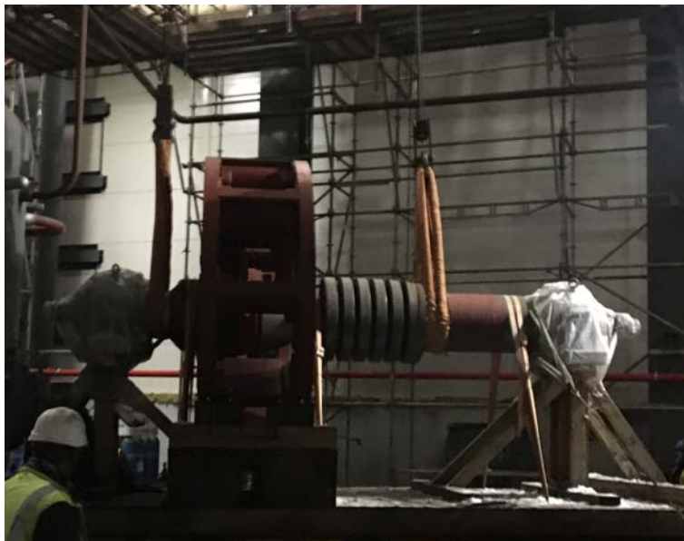
Example for lifting the rotor unit
