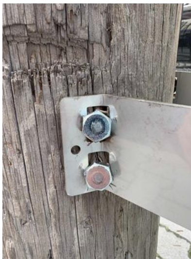
Figure 22 - Example of screws installed in wooden pole
