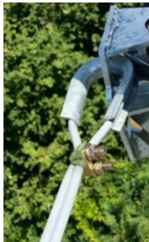
Figure 34 - Example of dielectric rope fixing to pole anchoring point
