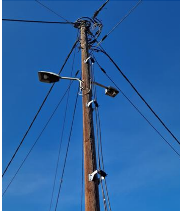
Figure 17 - Example of Cable pole distancecers installed on pole
