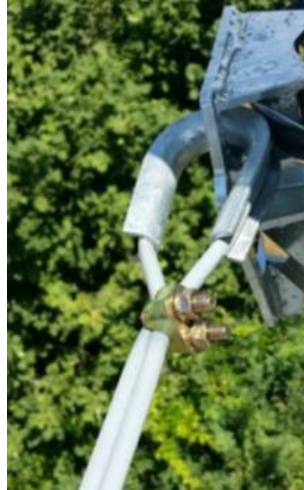
Figure 20 - Example of dielectric rope fixing to pole anchoring point
