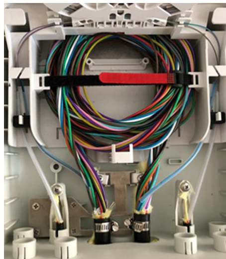
Figure 2 - Example of SDP midspan's uncut tubes management
