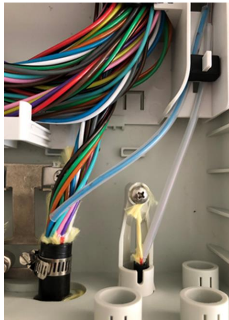
Figure 1 - Example of tubes routing inside SDP
