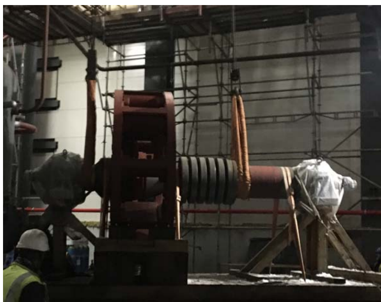
Example for lifting the rotor unit
