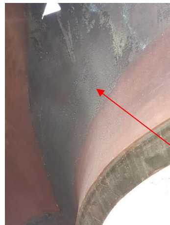
Missing TBC (post operation)
