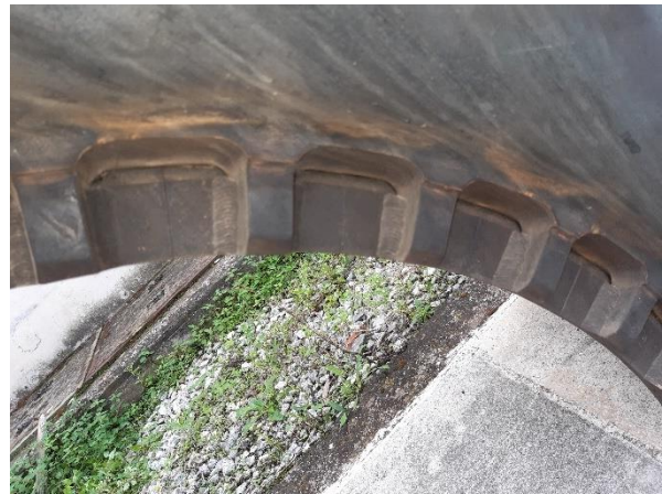
Compressor Suspension Ring – only light fretting contact surface
